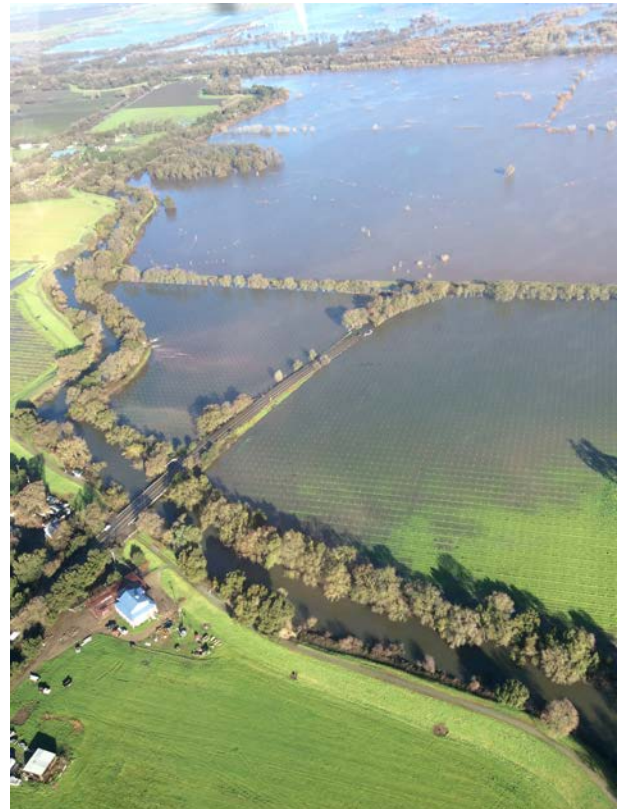
January 11, 2017 New Hope Levee Break
