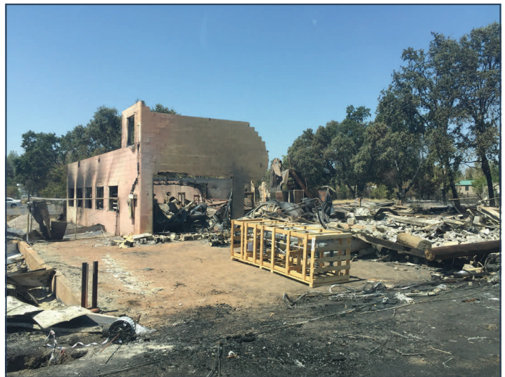
Fire damage to an historic structure from the Clayton Fire
