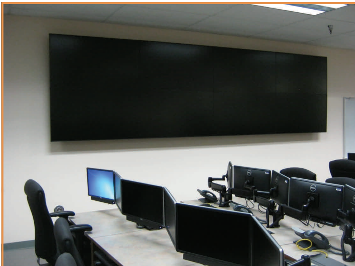
New 8-panel monitor wall
